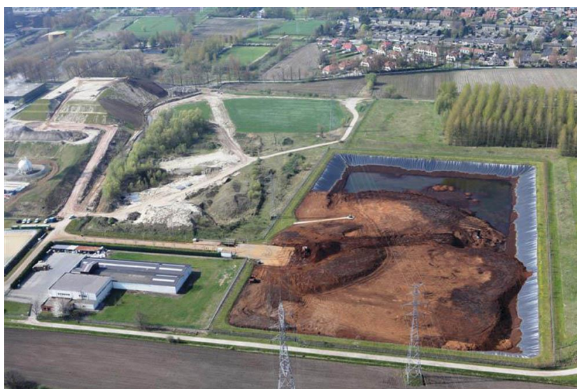
Figure 25: Covering landfills: capping of a landfill 31
