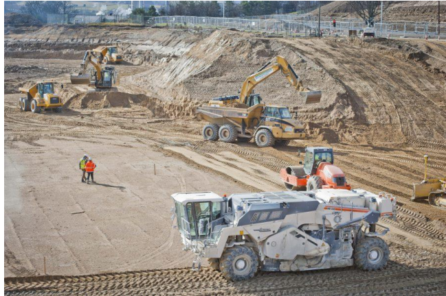
Figure 21 : Reclamation of excavated areas (in construction) - earthworks 27
