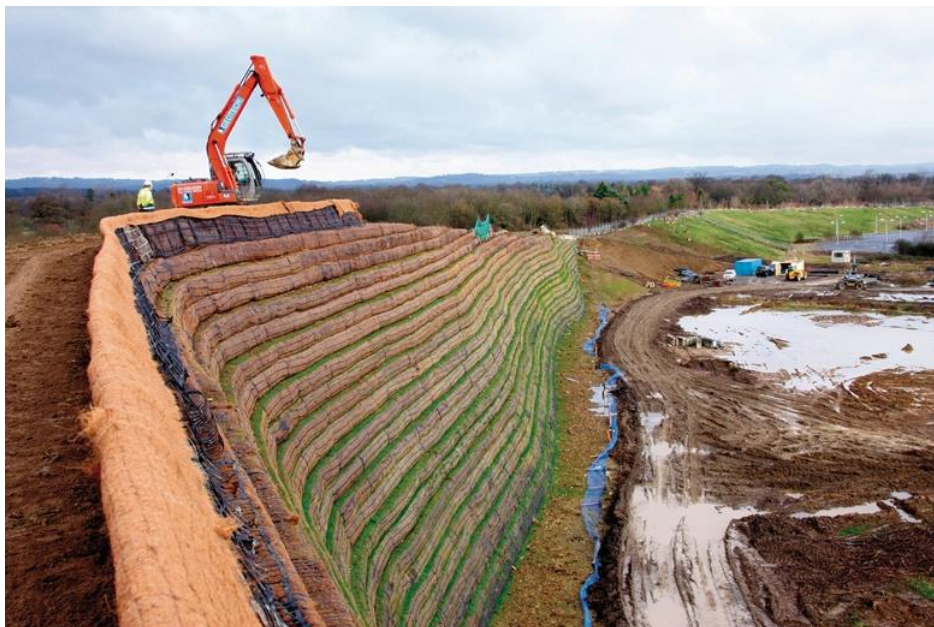
Figure 24: Landscape engineering: an example of a noise bund/barrier 30
