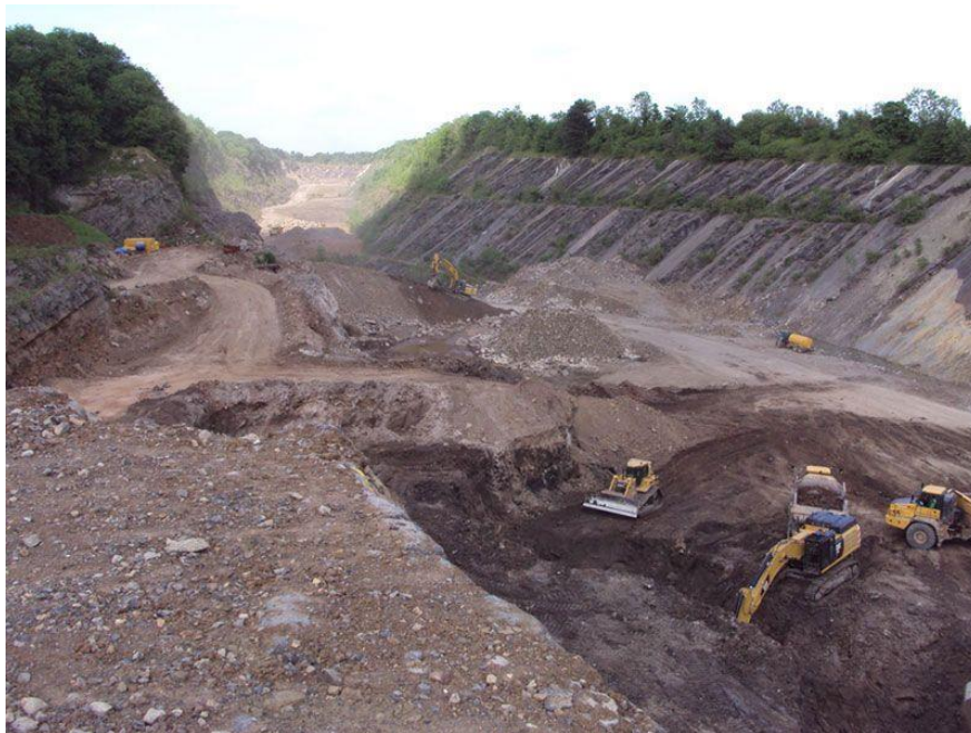
Figure 23: Reclamation of excavated areas: filling in a quarry void 29
